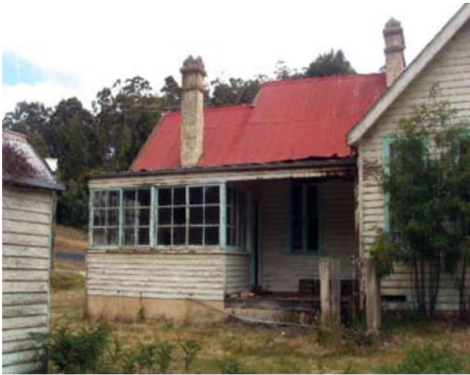
Woodsdale State School under renovation
