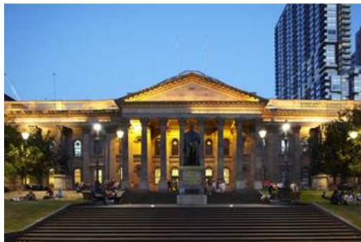
Photo: State Library Victoria facade (by Andrew Lloyd, courtesy State Library Victoria).
