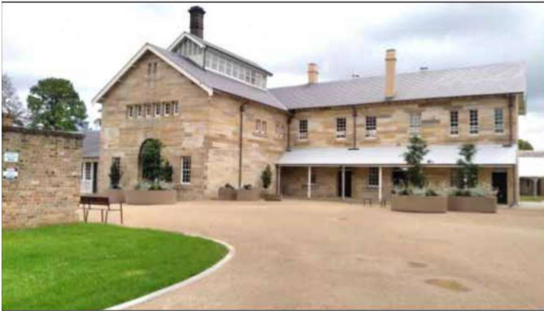
Left: The restored former Asylum Ward - entrance to the WSSH
