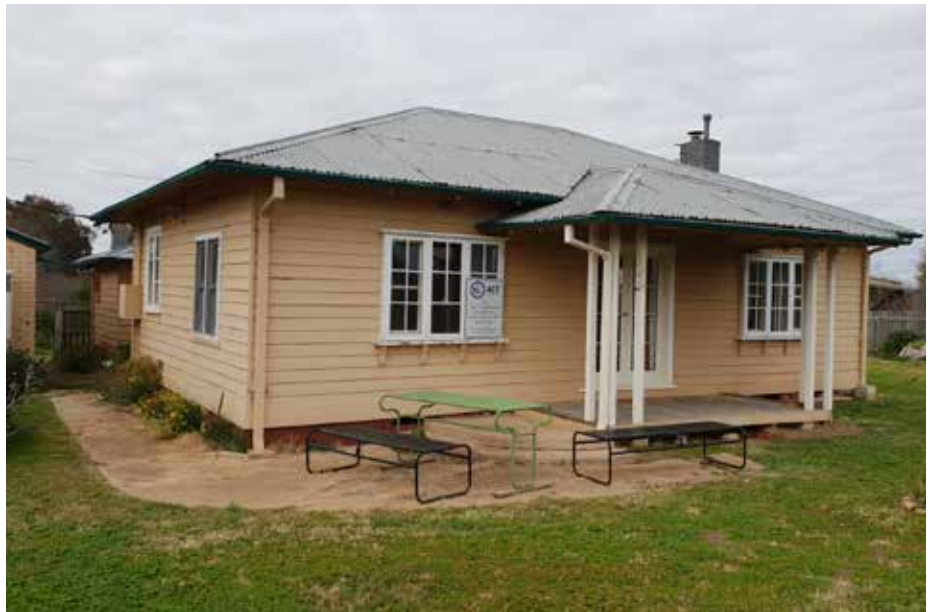
Cargill's Cottage. The Big Gun Dairy farmhouse.
