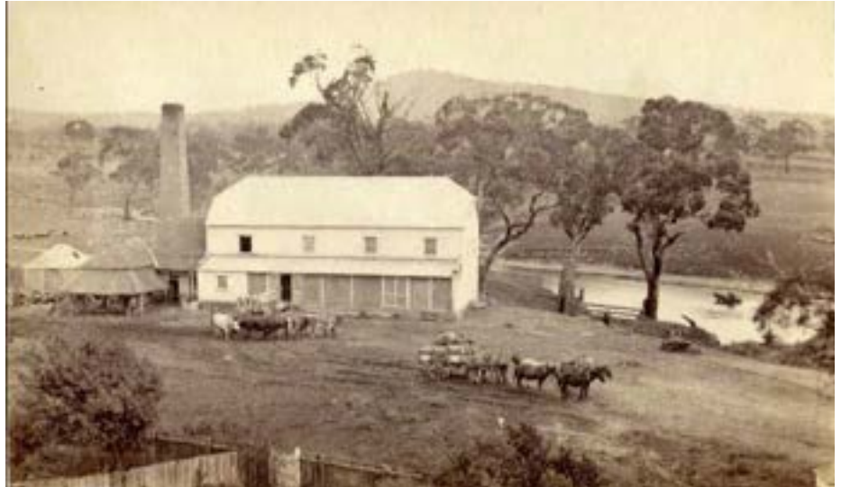
Loading at the Severne Mill on the Queanbeyan River, taken from Mill House. Beaufoy Merlin, 1870. CDHS collection.
